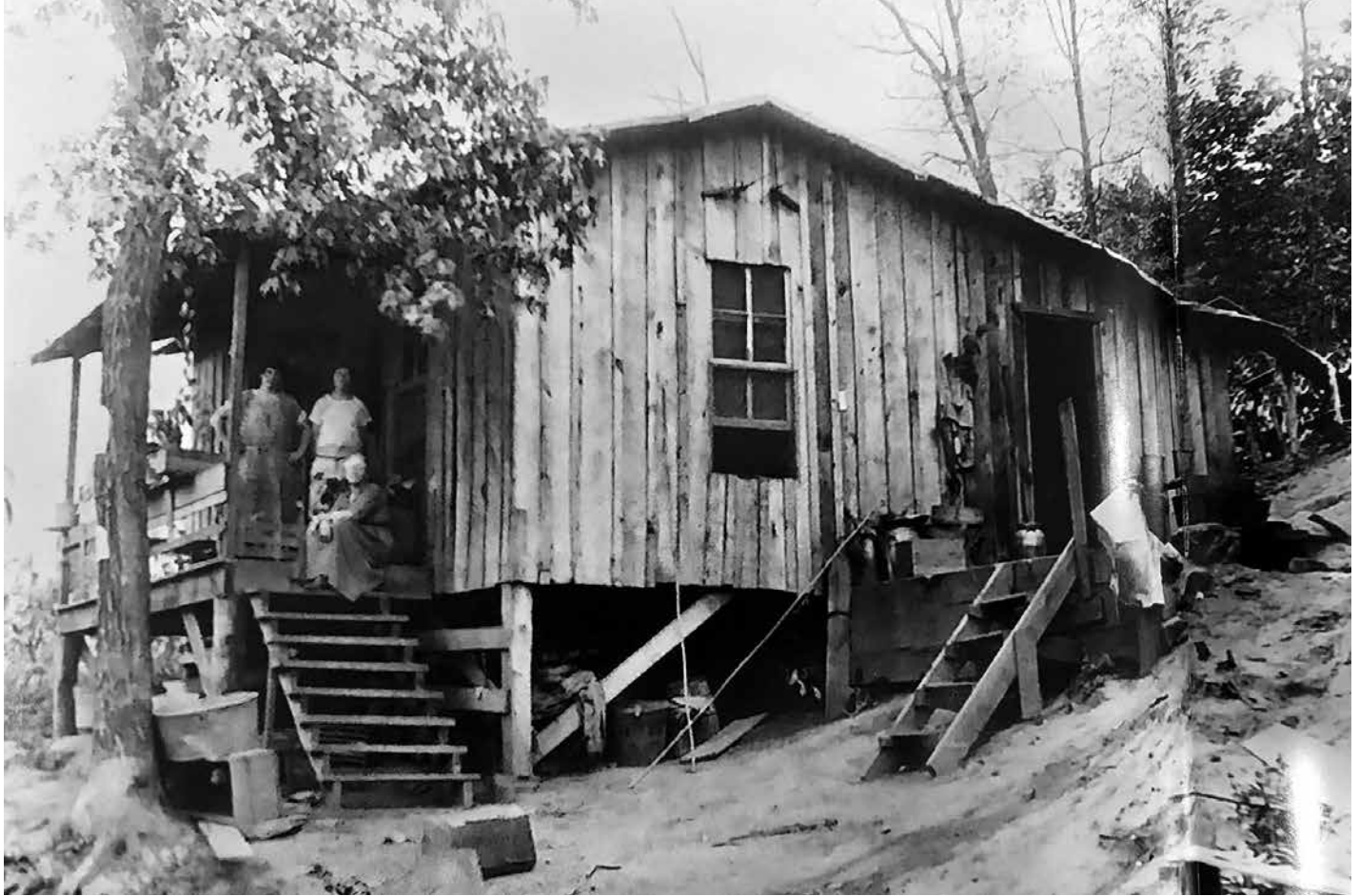
Cabins like this one housed dam workers during the construction.
