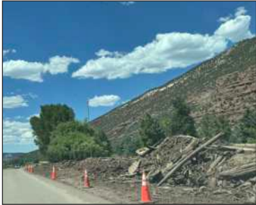
Photo by Katey Fetch The aftermath- a wall of debris along Highway 550 between Ouray and Ridgway
