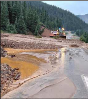
photo by CDOT Cleanup was a big task for CDOT with 8 mudslides between Silverton and Ouray
