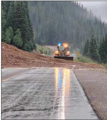
photo by CDOT Mudslide on Highway 550 near Chattanooga curve after the torrential rains last week
