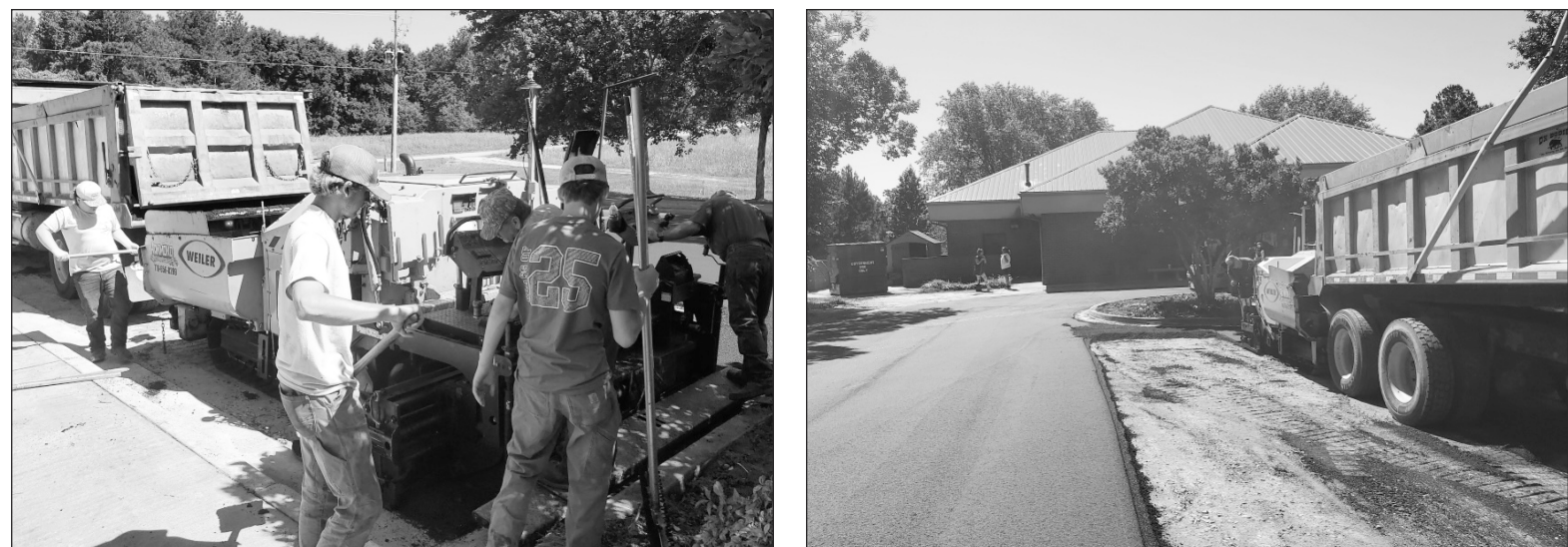
Workers repaved and added 16 more spaces to the Oglethorpe County Senior Center parking lot last week. The center averages 47 clients a day, but had only 22 parking spaces, forcing members to park along the side of the road or in grassy areas. The project was approved by the Oglethorpe County Board of Commissioners during its May meeting and completed last week.
