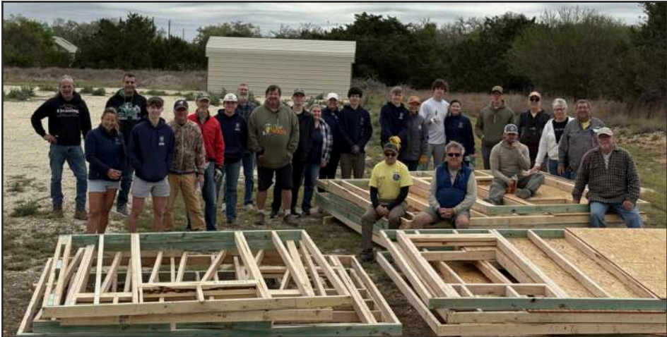
Volunteers constructed the walls for Melody Snell’s new home offsite at Dripping Springs Presbyterian Church, with help from the DS Young Men’s Service League.
