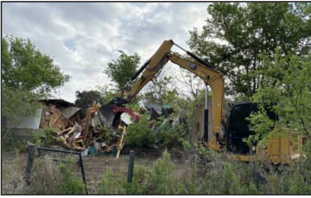
Sunset Construction and Excavation was in charge of the demolition on March 30.
