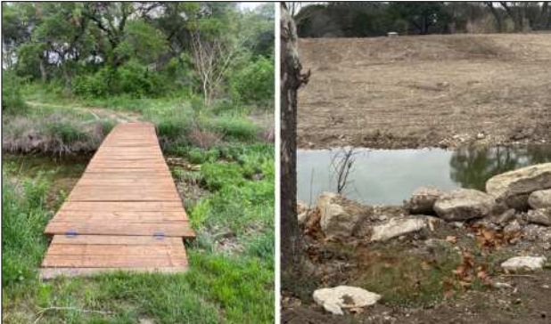
A footbridge on the Gestner farm is shown before and after the flood. PHOTOS COURTESY OF GREGG GESTNER.
