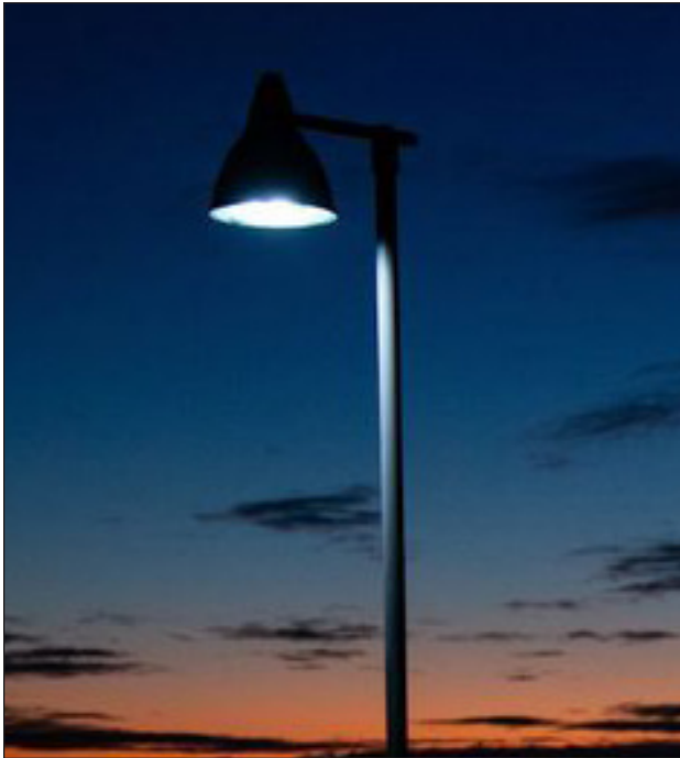
Shielded, downward-facing light fixtures help direct light where it is needed and prevent it from spilling into the night sky or neighboring properties. PHOTO COURTESY OF DARK SKY TEXAS
